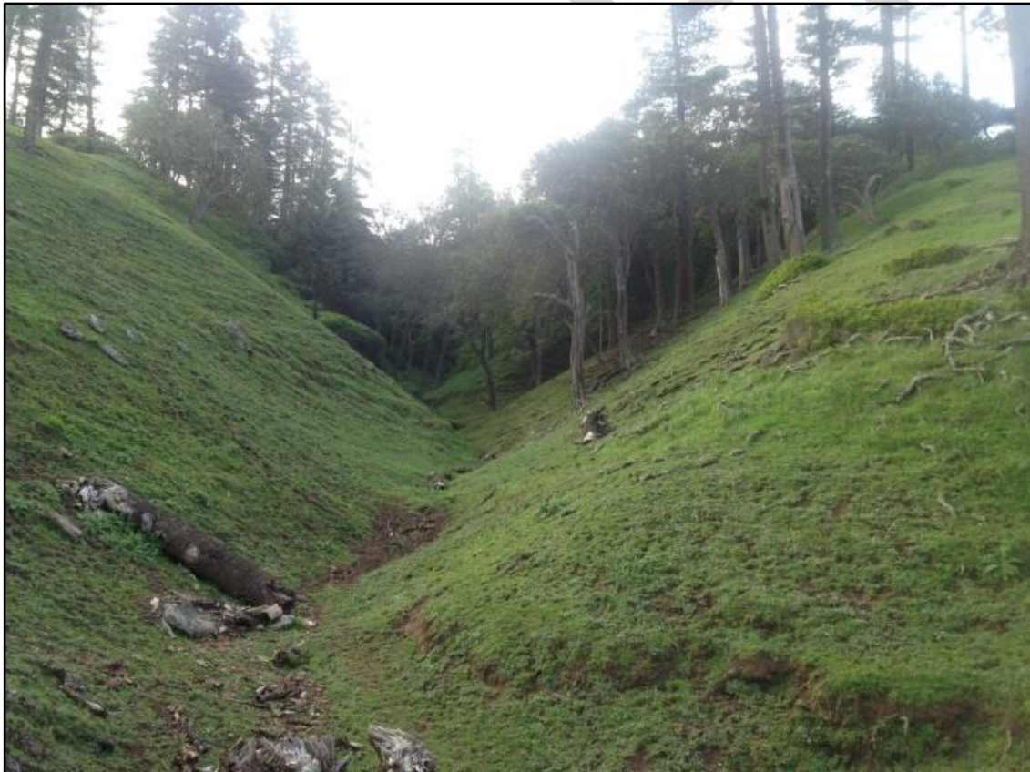
Figure 4. 2017 photo of cleared, grazed steep slopes. Despite recent rain and grass cover, exposed tree roots are visible, and terracettes can still be seen along the slopes
