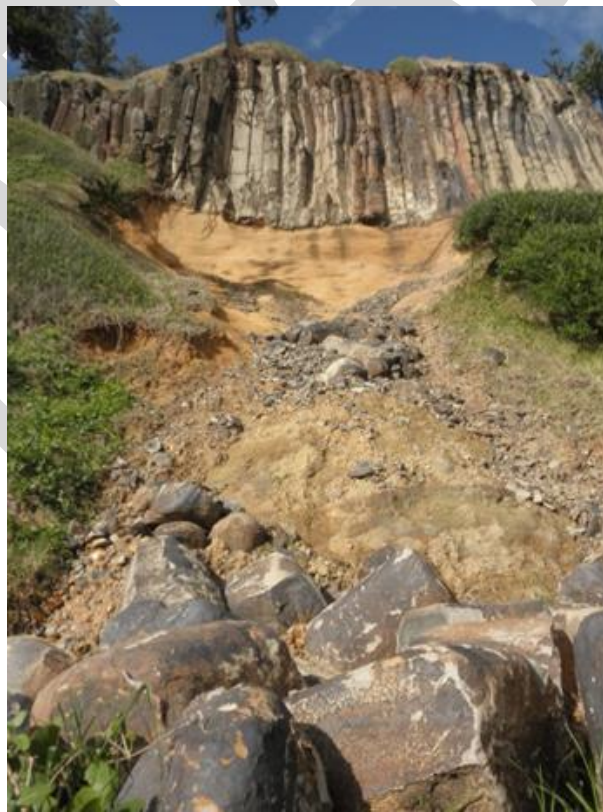
Figure 9: Rockfall from columnar basalt cliff above beach access track.
