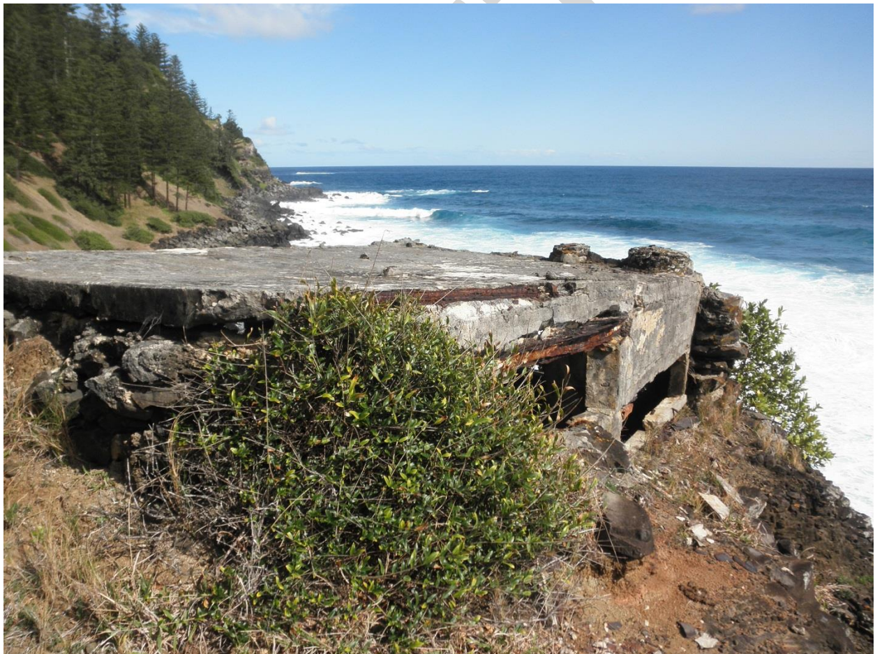
Figure 6: WWII Machine Gun Post, looking towards Selwyn Reserve.
