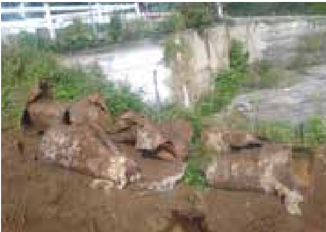
Out with the old - drums used as drains under the footpath, all clogged up with dirt.
